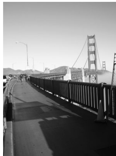
Exhibit 3-2 Bridge Sidewalk (eastside)
