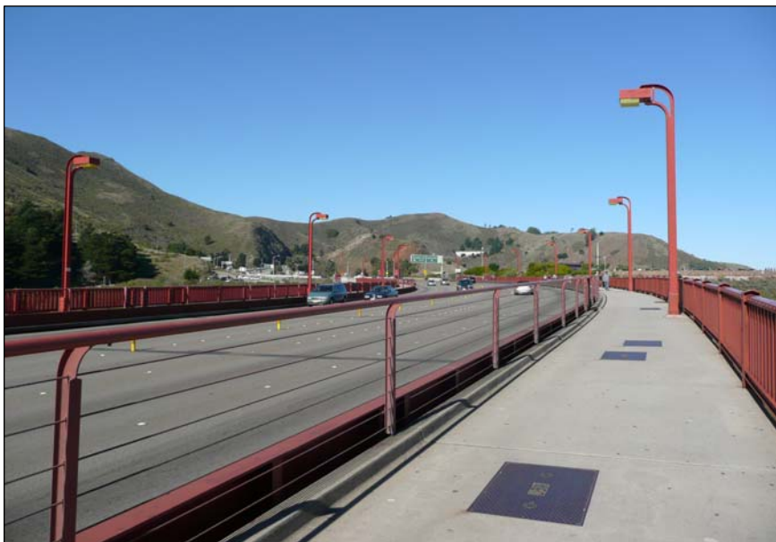
View of North Viaduct, showing public safety railing left of sidewalk, and existing railing right of sidewalk, camera facing north, November 2007. (Source: JRP Historical Consulting, LLC)
