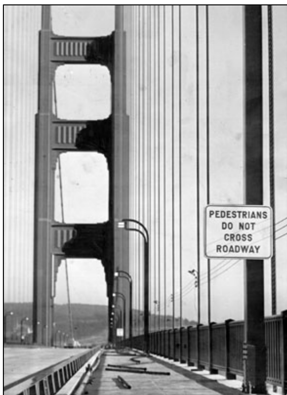
Photograph of sidewalk, railing, light standards and roadway, just days before the Bridge opened in May 1937, with original light fixtures. (Permission pending: San Francisco Historical Photograph Collection, San Francisco Public Library)
