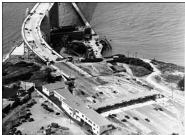
Detail of 1937 photograph showing Toll Plaza and bridge administration building during bridge construction, with west entrance to the Toll Plaza Undercrossing (34 0069) visible underneath the southern end of the building. (Permission pending: San Francisco Historical Photograph Collection, San Francisco Public Library)
