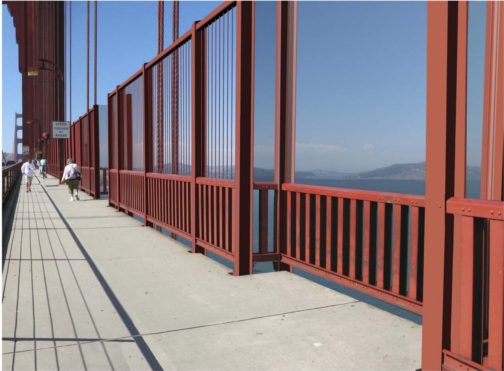
SIDEWALK NORTH 1A
