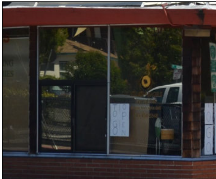
Figure 3. View of primary (west) façade, showing slider window, facing east. Source: ICF 8/11/2020.
