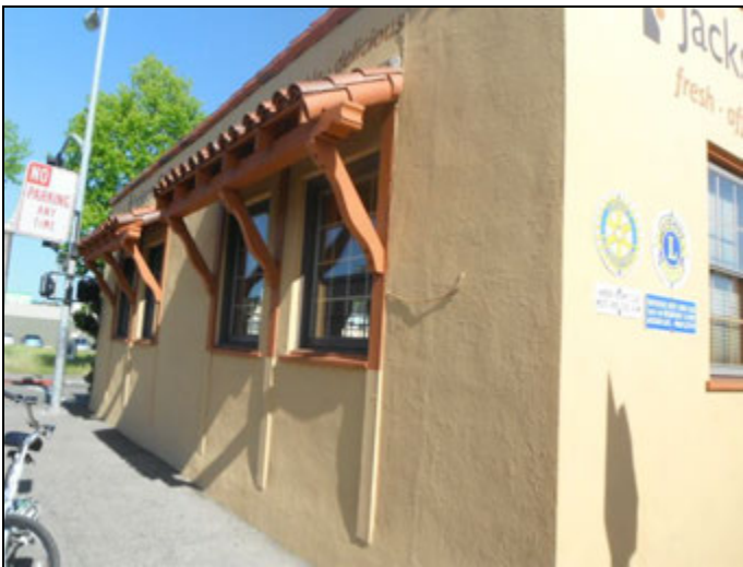
Photograph 5. Northwestern Pacific Depot. 930 Tamalpais Ave. View northwest.
