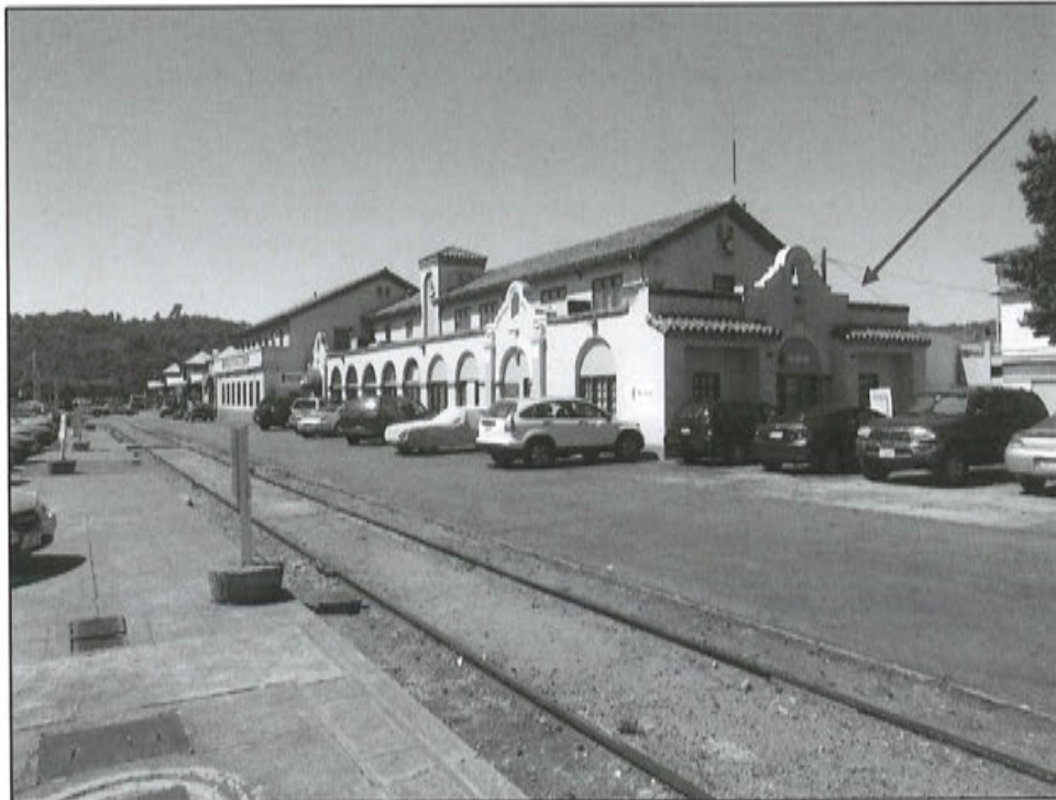
Photograph 2: North end of building (indicated by red arrow) is an addition constructed in 1987 (see red arrow below indicating original design of north end). Row of arches at left was originally an open arcade. Camera facing southwest.
