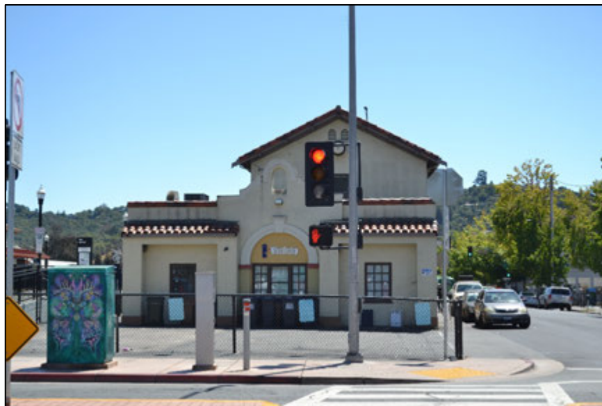
Figure 7. The c.1970s north addition, which replaced an earlier north addition dating to the 1950s (outlined in yellow in Figure 6 above). Viewed facing south.
