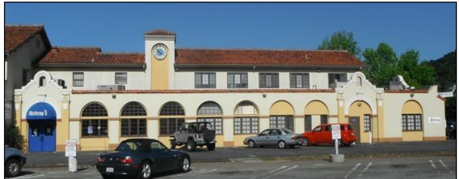
Photograph 2. East elevation of San Rafael depot showing infill of the arched arcade and an addition at the north end. Photograph taken on April 22, 2013.
