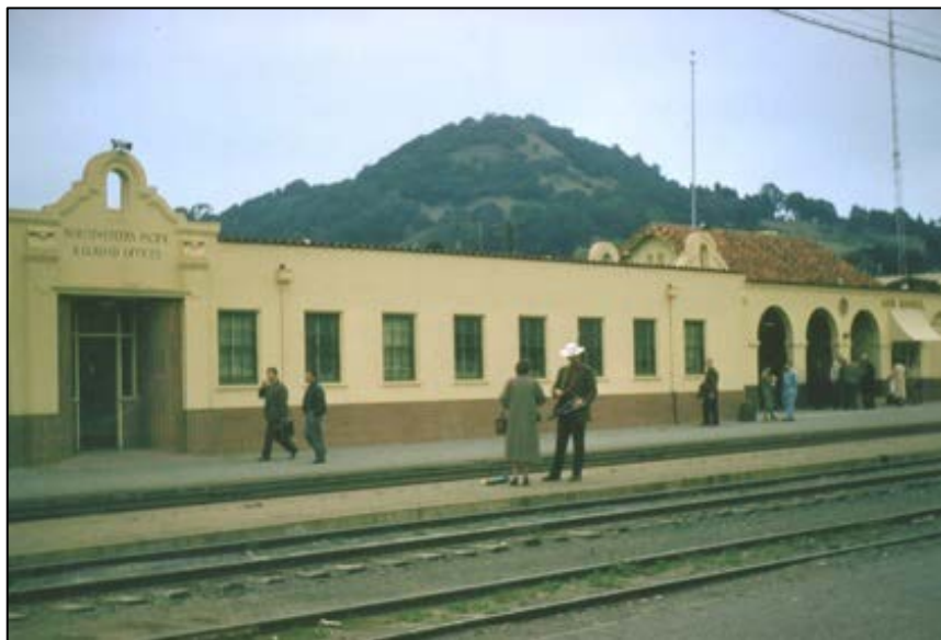
Figure 5. Depot building, viewed facing northwest, shows the c.1940s NWP office addition, which blocked the south end of the passenger arcade. The northernmost arches in the arcade had also been enclosed at this time (at far right of image). Source: Anne T. Kent California Room, Marin County Free Library, via San Rafael Heritage.
