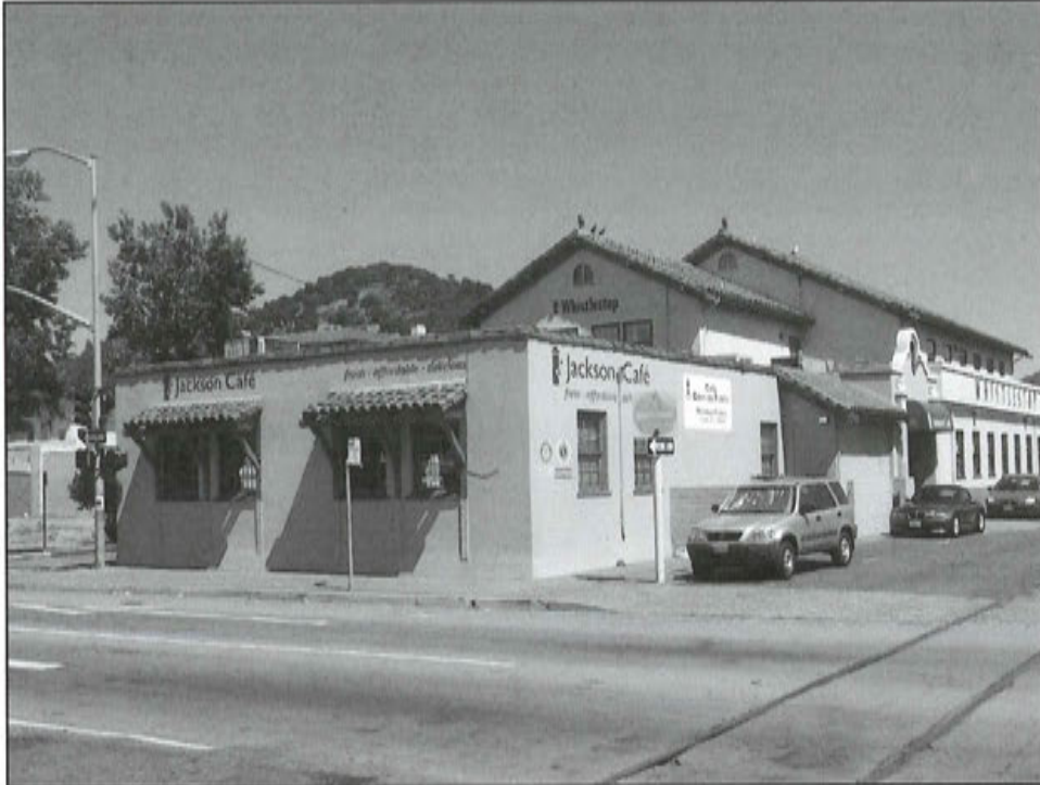
Photograph 7: South end of building, camera facing northwest.
