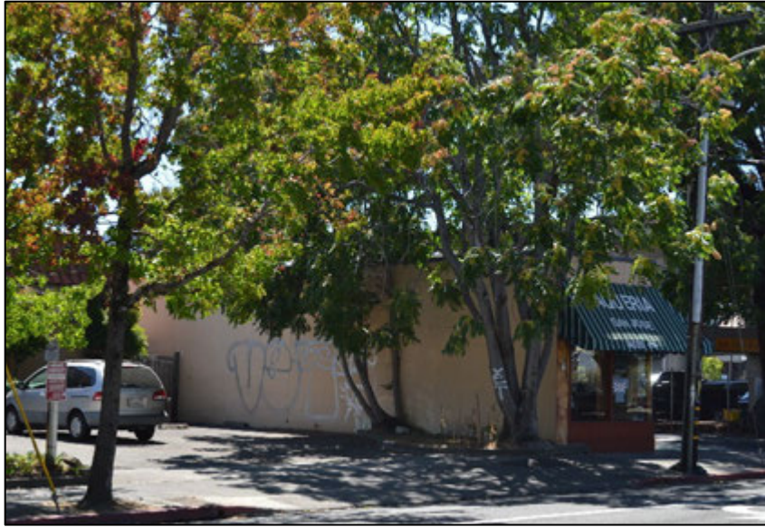
Figure 2. View of primary (north) and east façades, facing southwest. Source: ICF 8/11/2020.
