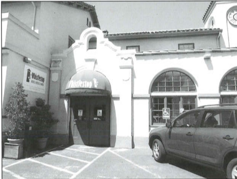
Photograph 9: Entry at south end of former arcade on east side, camera facing west.
