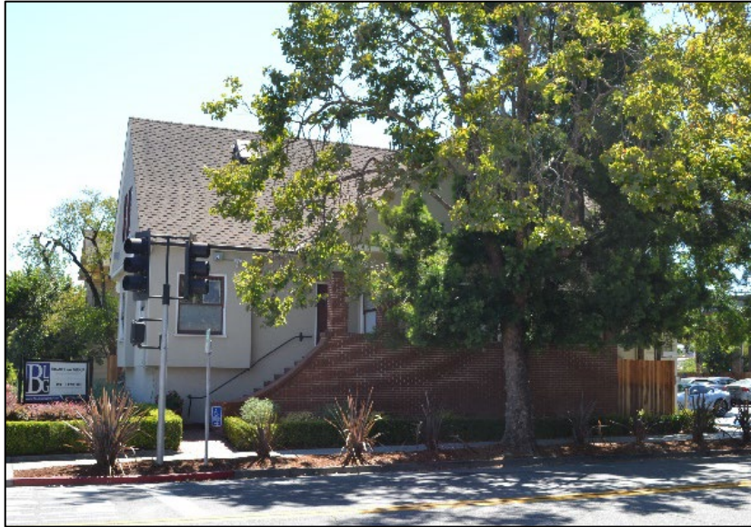
Figure 2. View of the primary (north) façade, facing south. Source: ICF 8/11/2020.
