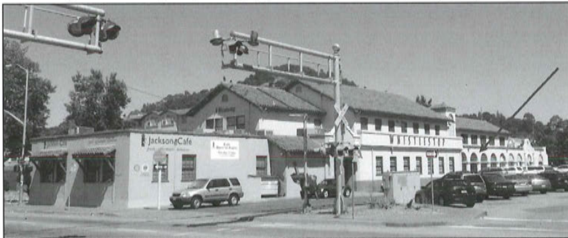
Figure 3: Former San Rafael Depot, July 31, 2012, camera facing northwest. Note extensive additions to the second story, enclosed arcade at right, and additions to south end at left.
