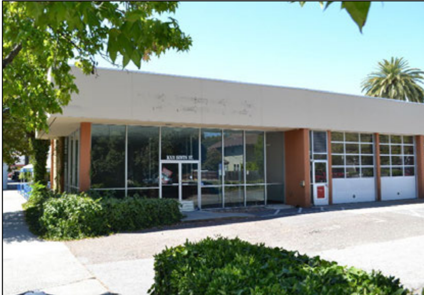
Figure 4. View of the south end of the primary façade, facing west, showing the showroom and main entrance. Source: ICF 8/11/2020.
