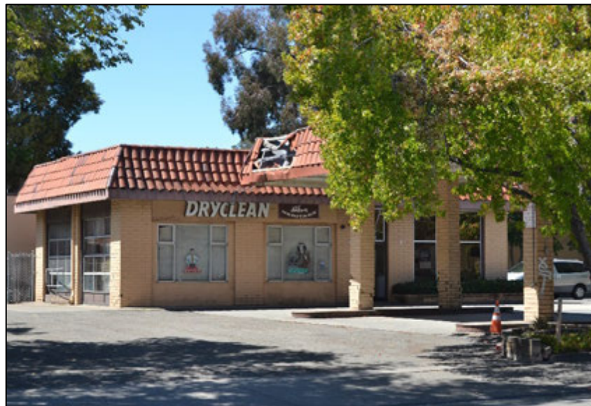
Figure 3. View of primary (east) and south façades, facing northwest. Source: ICF 8/11/2020.
