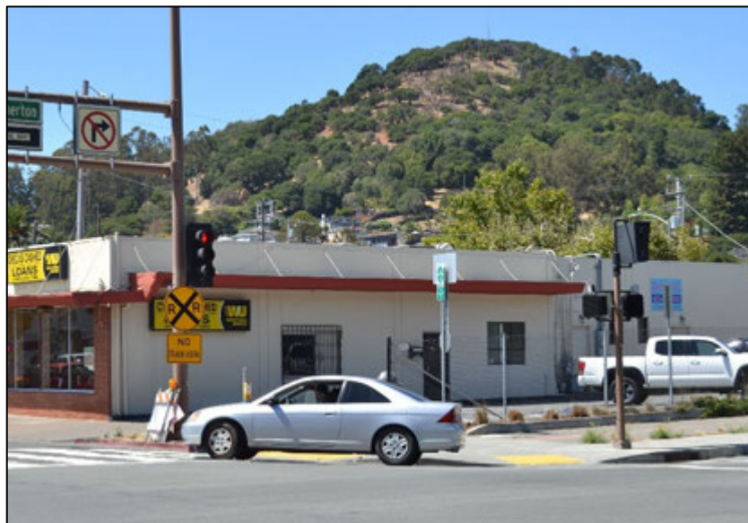
Figure 5. View of east façade, facing northwest. Source: ICF 8/11/2020.
