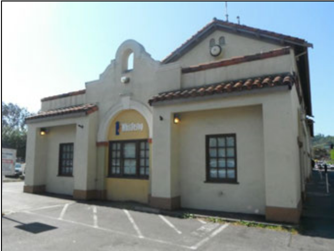
Photograph 3. Northwestern Pacific Depot. 930 Tamalpais Ave. View south.
