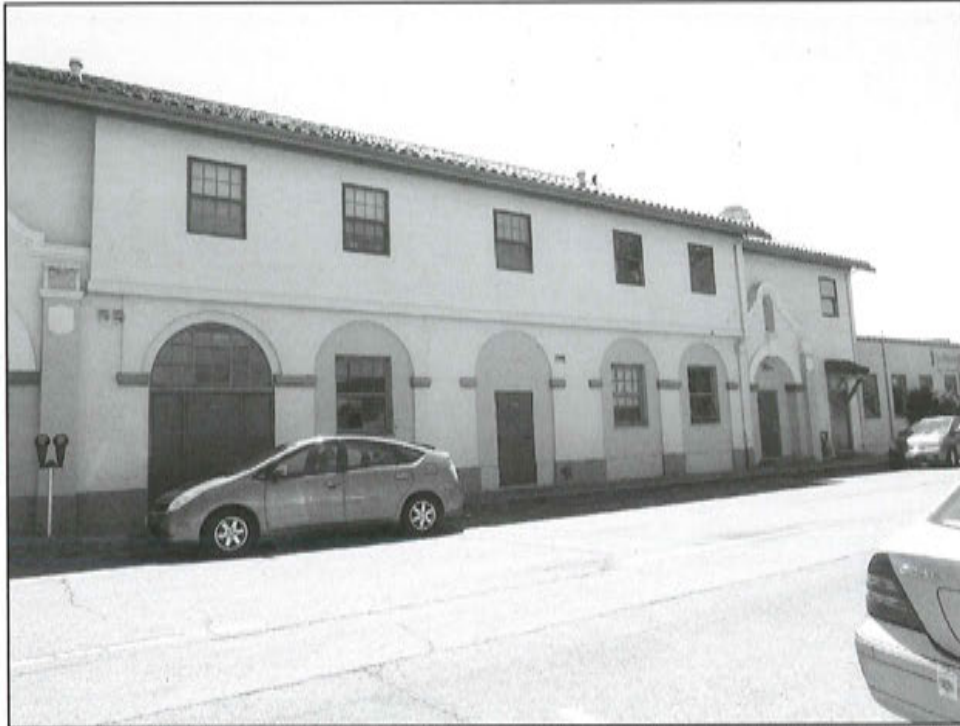
Photograph 5: West side showing 1985 second-story addition, camera facing southeast. Also note various treatments of ground-level arches.
