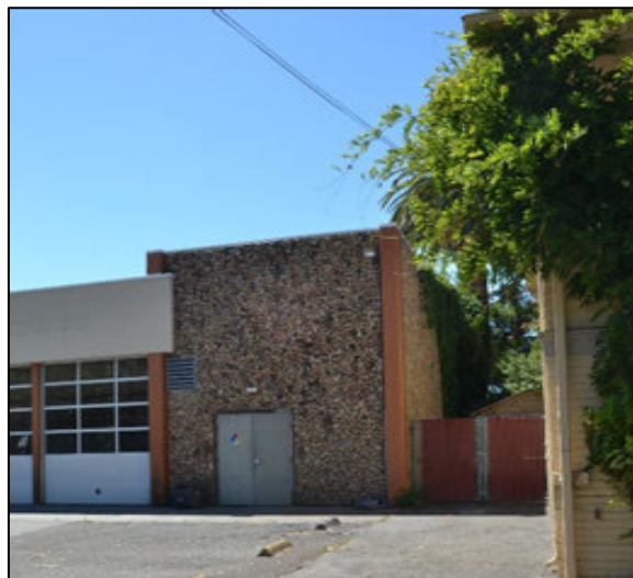
Figure 5. View of north end of primary façade and north façade, facing west, showing the stone veneer cladding at the building's north end. Source: ICF 8/11/2020.
